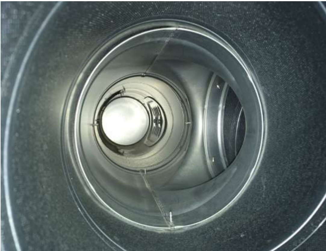
DUCTWORK AFTER CLEANING
