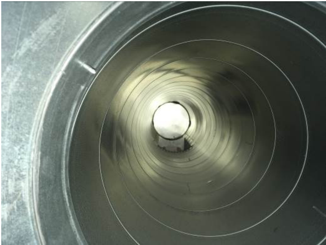
DUCTWORK AFTER CLEANING
