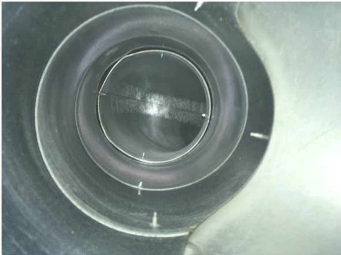
DUCTWORK AFTER CLEANING
